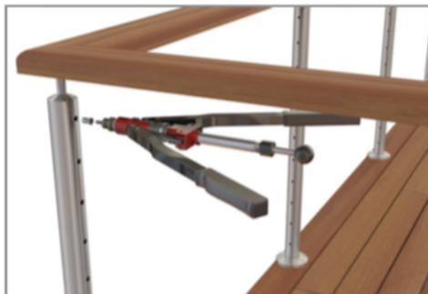
Use the HN-02 nut rivet tool to insert all left hand nut rivets into left hand post and all right hand nut rivets into right hand end post.
