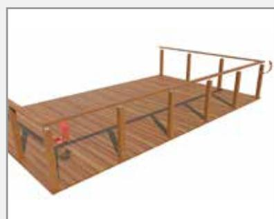
Tension both ends of the wires evenly, rotating the wire in the same direction, using the ProRig c-spanner. **Note:** You may require a person at each end of the wire to tension effectively.
