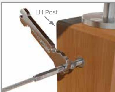
Make sure the left hand swage stud is wound into the left hand threaded insert, only screw the swage stud into the threaded insert the minimum amount possible for wire to hold.
