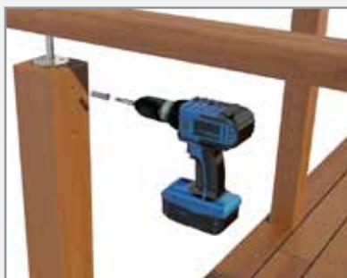
Use the 6mm hex drive bit to screw the threaded inserts into the pre-drilled end posts. **Note:** Insert all left hand threaded inserts into left hand post and all right hand threaded inserts into right hand post.
