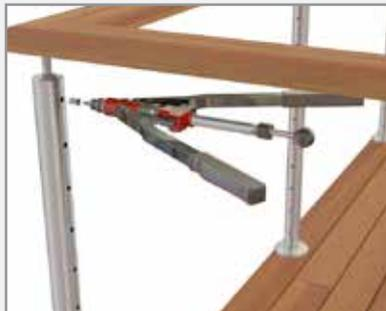
Use the HN-02 nut rivet tool to insert the nut rivets into the pre-drilled posts. **Note:** Insert all left hand nut rivets into left hand end post and all right hand nut rivets into right hand end post.
