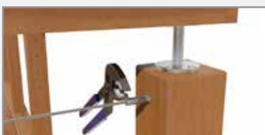
To lock the system in place, tighten the finishing cap against the head of threaded insert using the PL-10 soft jaw pliers.
