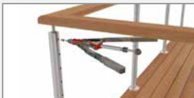
Use the HN-02 nut rivet tool to insert the nut rivets into the pre-drilled end posts.
